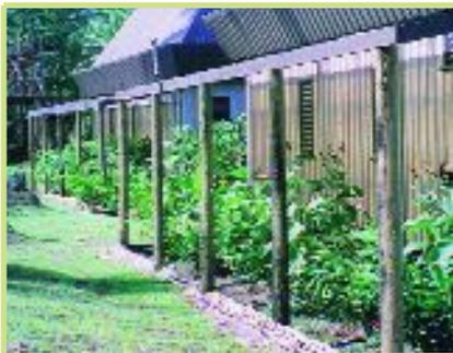
The owners of Lalati, a resort on Bega island, Fiji, wanted a wastewater system that would not pollute the water. Ecological Engineering Group designed garden-like wastewater systems that use up wastewater at each building. The system also features site-built composting toilets with micro-flush toilets that are compatible with an upscale resort. Guests feel good knowing they are not polluting the island's coral reefs which provide world-class diving.
